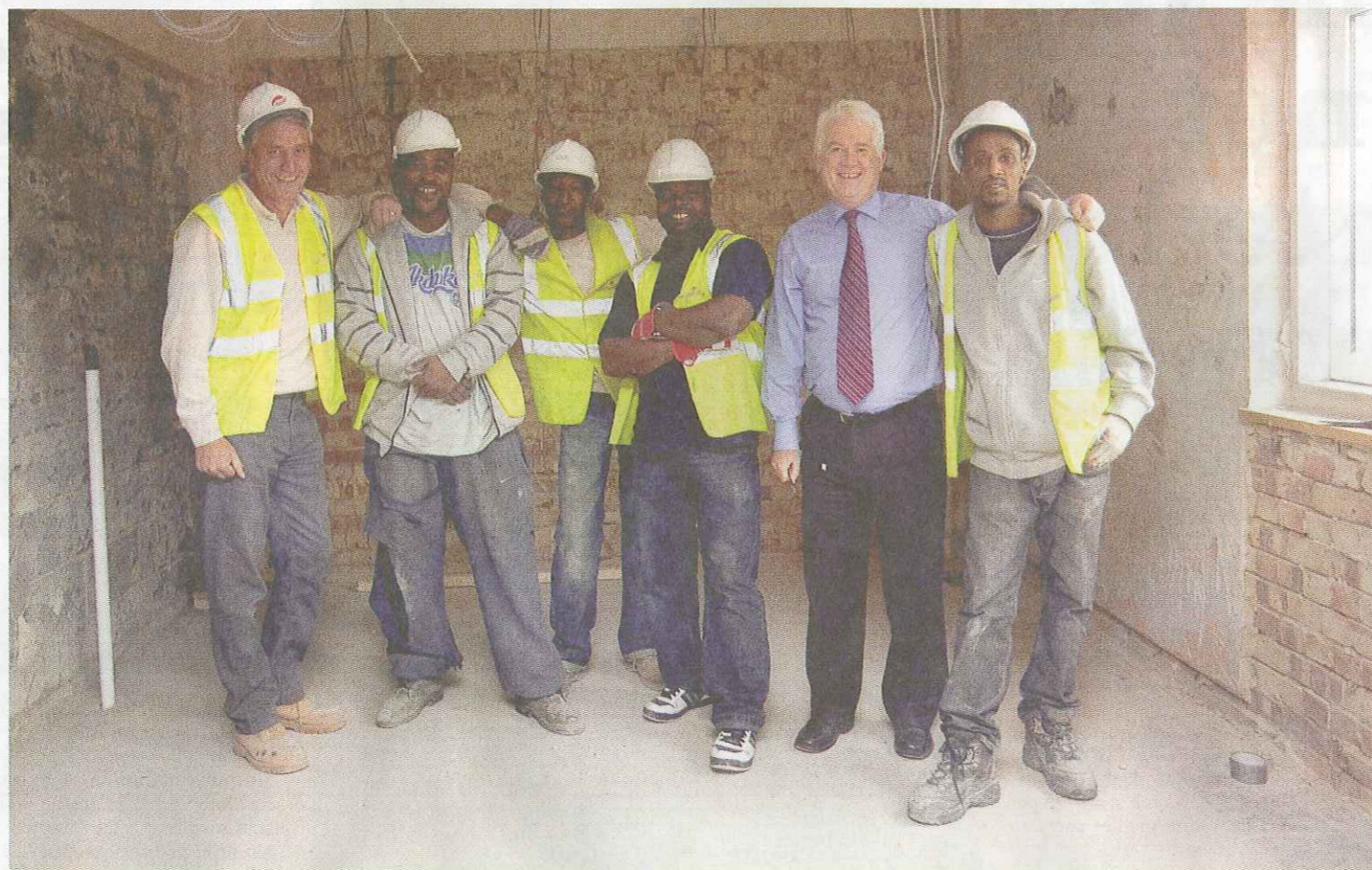
Director Keith Fernett with 4 residents who have been employed by our contractor to rebuild Anchor House
